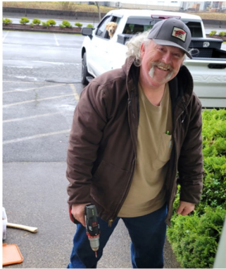
David Cox works to reinforce the wooden frame.
